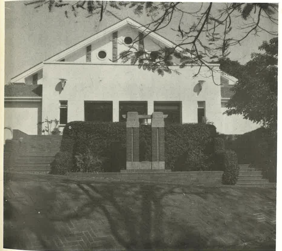
The facade of the School Hall - G. Johnson.
